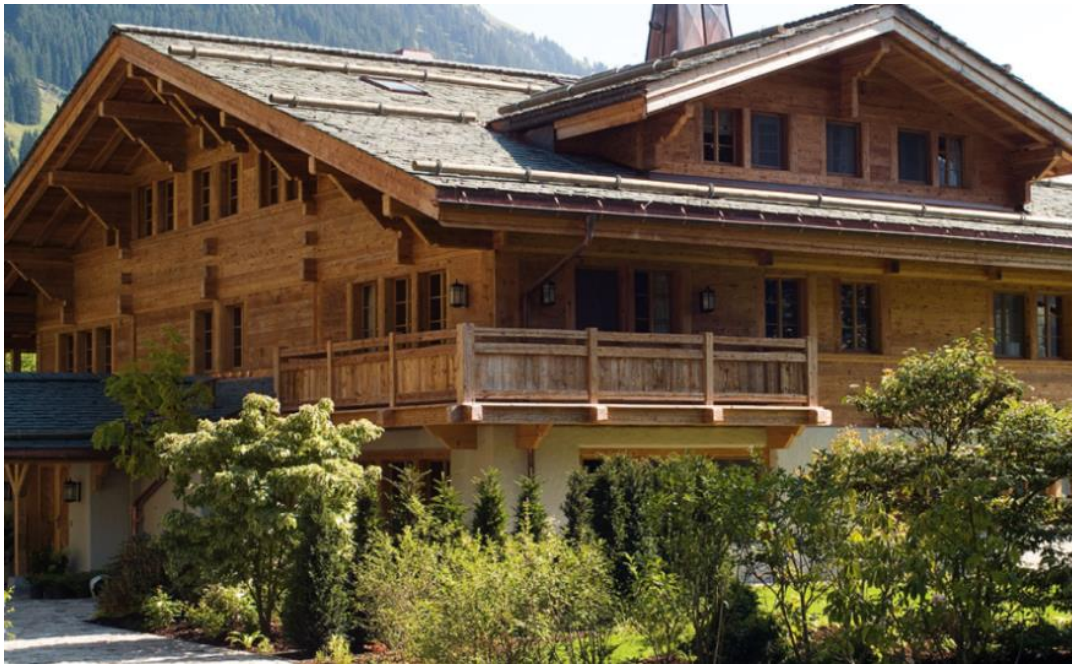
New building with 200 years old wood (Chaletbau Matti/CH)
