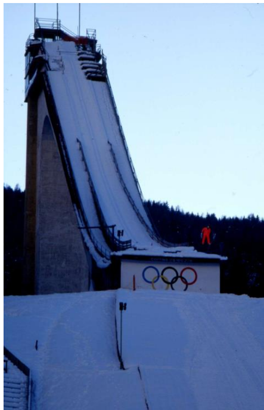
FIGURE 23.2 The ski jumping trampoline of Cortina d'Ampezzo, Italy, used during the 1956 winter Olympics. The inrun was covered by timber boards, in turn covered with snow and ice. Disused since 1990, today it remains a relevant historical monument (image courtesy of Servizi Ampezzo Unipersonale S.r.l.).
