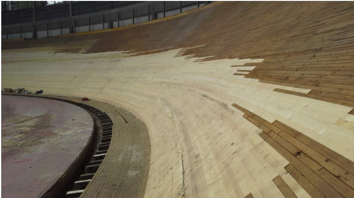
FIGURE 31.2 During the restoration of the Vigorelli velodrome track, around 20% of the boards were replaced and the remaining wooden elements were restored (image A. Galbiati).
