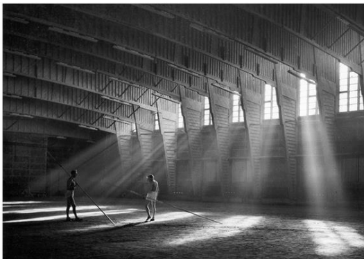
FIGURE 5.1 For the Olympic Games Helsinki 1952, Alvar Aalto (Reed 2009) designed a sports center in Otaniemi (Espoo, Helsinki) - today still perfectly operational - which impresses with the simplicity and elegance of its wooden structures, representing an extraordinary example of technological innovation in wooden construction of that time. Made of thin prefabricated timber trusses (Isohauta 2013), the structural "skeleton" can be considered a demonstration of architects and engineers' ability to experiment innovative constructive systems starting from new wood-processing industry construction products. Photograph copyright: Museum of Finnish Architecture, Heikki Havas.
