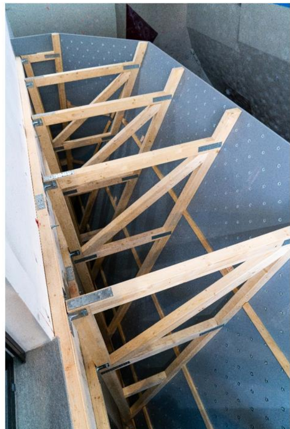
FIGURE 27.2 Left: An artificial climbing structure (ACS), equipped with resin holds and fixed quickdraws [photo courtesy of Sint Roc S.r.l., Arco, Italy]. Right: An ACS supporting frame made of glue laminated timber (glulam) [photo courtesy of Explore Climbing s.n.c., Tonco, Italy].
