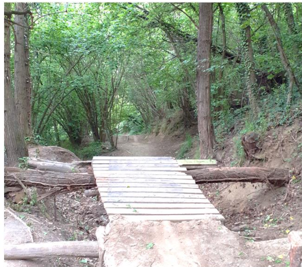
FIGURE 20.1 Left: timber boardwalk installed in a downhill track in a mountain larch wood (image F. Negro). Right: jump in a downhill track, made of timber boards mounted on a frame fixed to horizontal logs (image F. Negro).
