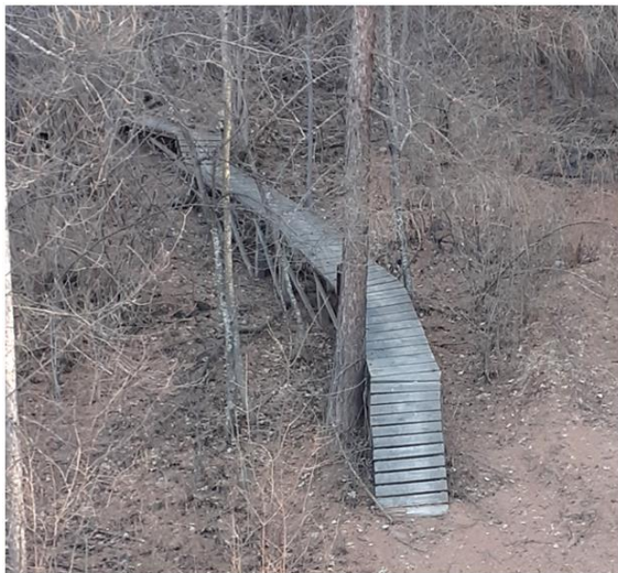
FIGURE 20.1 Left: timber boardwalk installed in a downhill track in a mountain larch wood (image F. Negro). Right: jump in a downhill track, made of timber boards mounted on a frame fixed to horizontal logs (image F. Negro).
