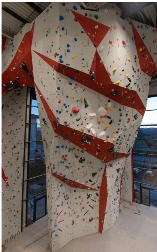
FIGURE 27.2 Left: An artificial climbing structure (ACS), equipped with resin holds and fixed quickdraws [photo courtesy of Sint Roc S.r.l., Arco, Italy]. Right: An ACS supporting frame made of glue laminated timber (glulam) [photo courtesy of Explore Climbing s.n.c., Tonco, Italy].
