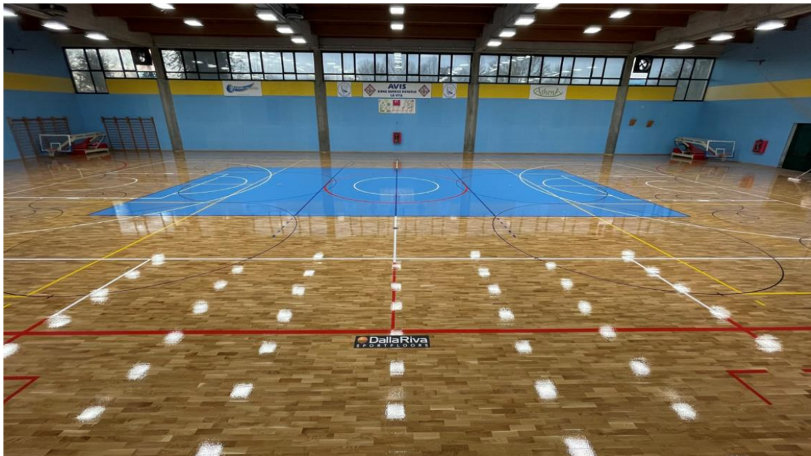
FIGURE 17.5 Oak wood floor with marking related to multiple sports (image courtesy of Dalla Riva Sport-floors).
