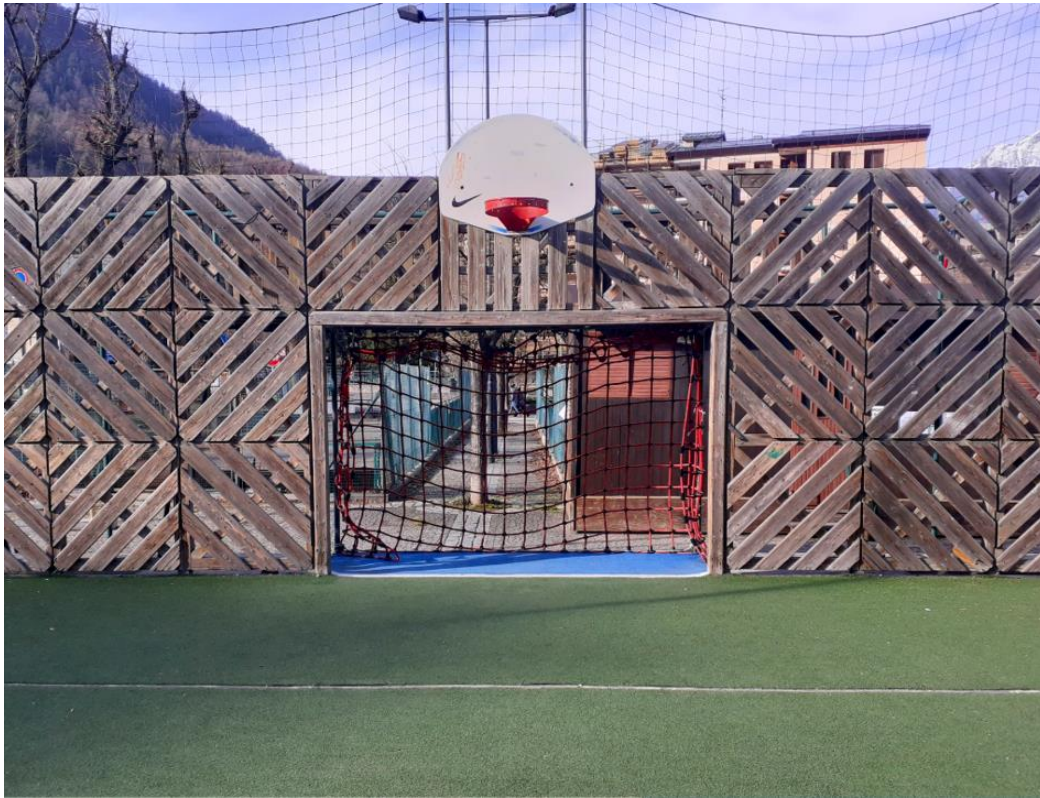
FIGURE 17.6 Timber elements of this outdoor, multi-purpose playing field (Oulx, Italy) perform different functions at the same time: they delimit the playing area, withstand the repeated impacts of the ball, and are key to determine the aesthetic appearance of the facility (image F. Negro).
