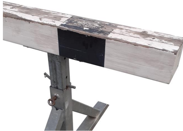
FIGURE 23.1 The shabby painting of this steeplechase hurdle clearly shows the laminate timber structure of the bar and is also a reminder of the need for regular maintenance of wood exposed to outdoor environments (image F. Negro).
