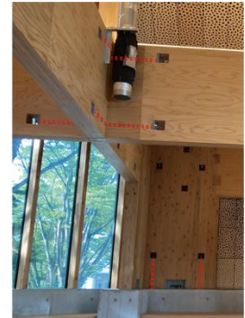
Figure 1. Tensile-bolted joints in building
